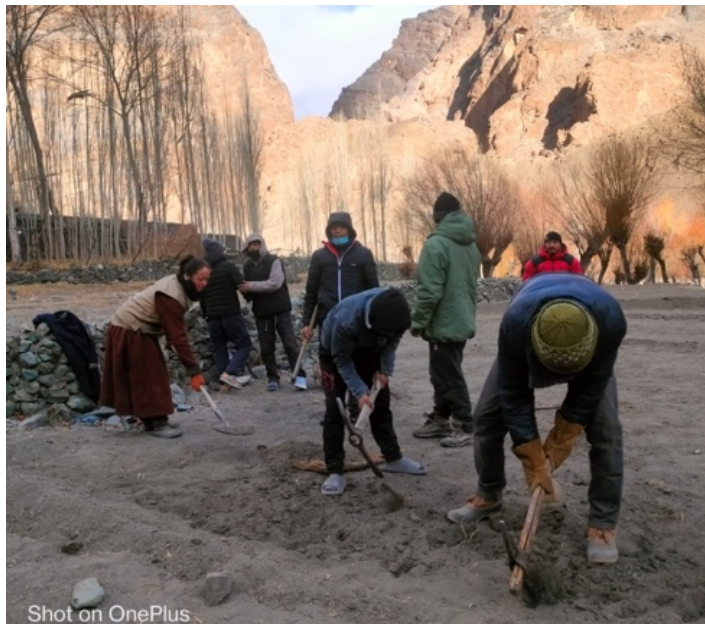
Leveling the site
